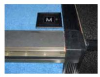
The crimped connectors should be inserted into the cable management, and the endcap fixed into the step edging
