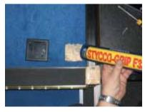
3. Use an adhesive suitable for the substrate
